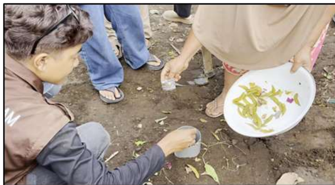
Gambar 4. Pengisian lubang Biopori
